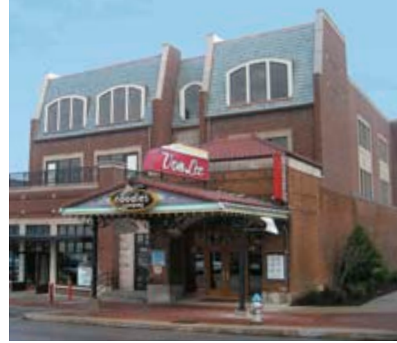
Chicago-based Tartan Realty Group redeveloped the historic Von Lee Theater near Indiana University in Bloomington, Ind., into retail and office space.
